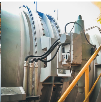
Butterfly Valve (32,000 Nm)
