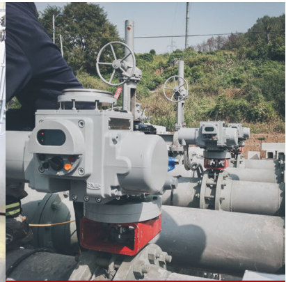
200A Butterfly Valve (1,100 Nm)
